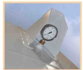
Canopy to Protect Pressure Gauge
